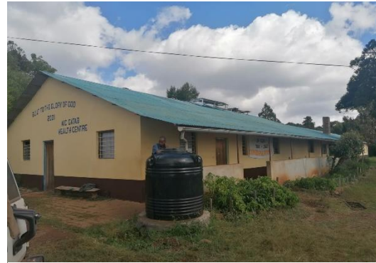
Plate 9. Community water point with water storage tank
